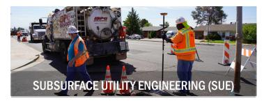
We identify underground utilities' location, depth, and characteristics as part of the design stage of constructing new infrastructure or placing new utilities. Utilizing SUE in the design stage helps eliminate project delays or redesign costs due to unforeseen utilities, avoids utility damage, and increases job site safety.
