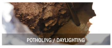
Hydrovac daylighting uncovers and exposes underground utilities, pipelines, and cables. Using our Hydrovac instead of hand digging or mechanical excavation reduces the risk of injury or damage to existing infrastructure. It carries a lower project cost, increases productivity, and improves project safety.
