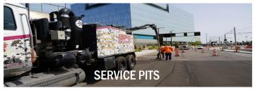
Repairs in developed urban areas do not always need manual excavation. Our skilled Hydrovac operators can excavate service repair pits, providing minimal disruption to existing infrastructure and allowing quick access to making repairs.
