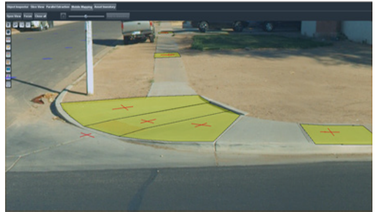
Ramp and Sidewalk features with running slope and cross slope lines.
